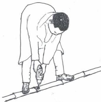
Figure 5: An illustration of drilling holes at alternate nodes
