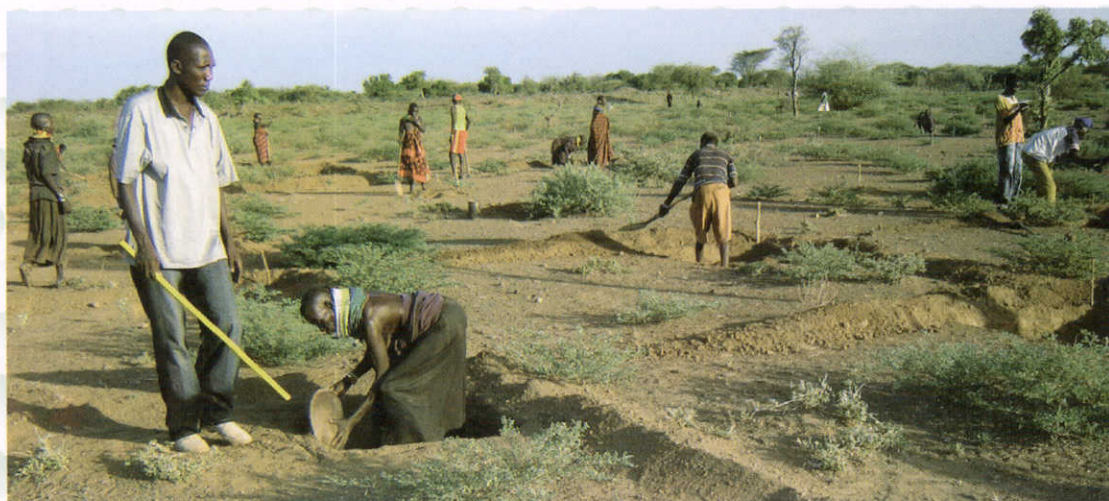
Preparation of micro-catchments at Pelekech
