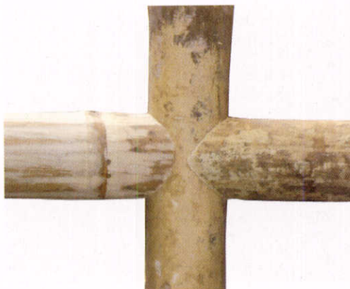
Samples of fish mouth joints
