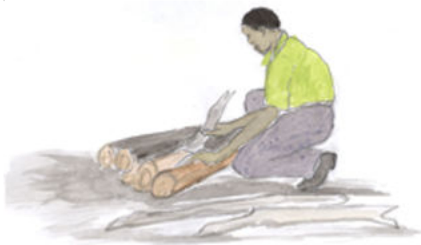
Figure 1: Debarking the crosscut posts
