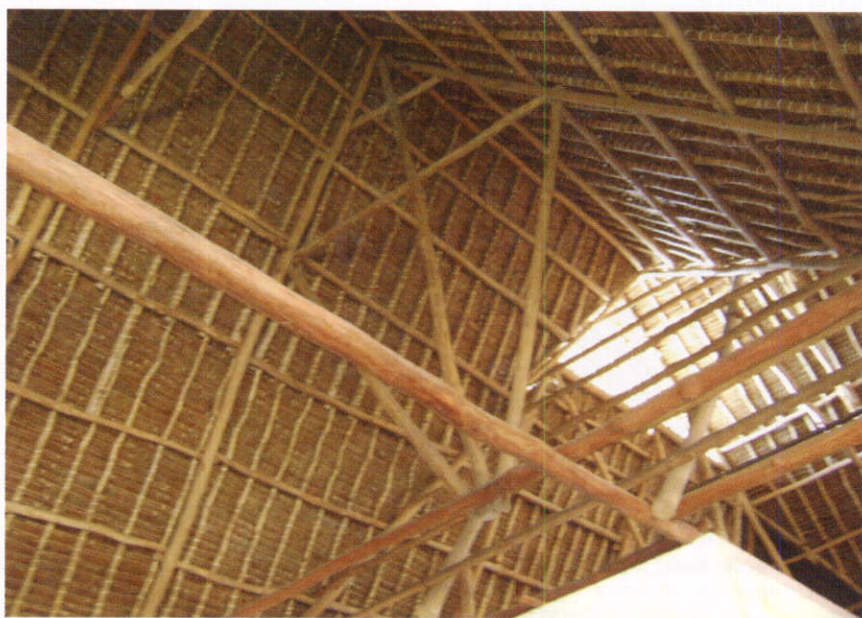
The poles are used for construction in the hotel industry. (Photo KEFRI)
