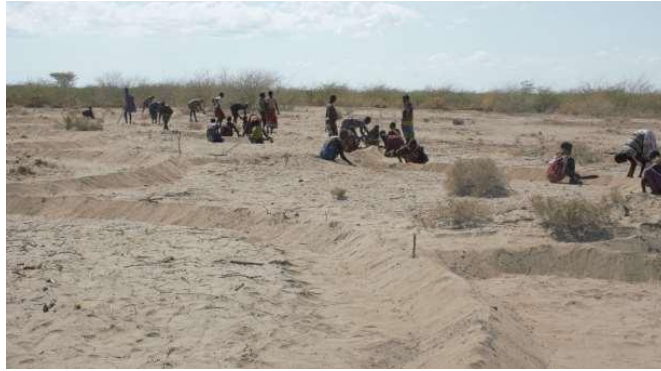
Figure 2: Community constructing micro-catchments in the area cleared off Prosopis (in the background) doing this by themselves after training was done.
